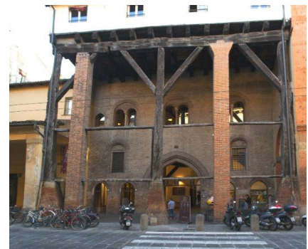
Figure 35; Portico with the three arrows.
