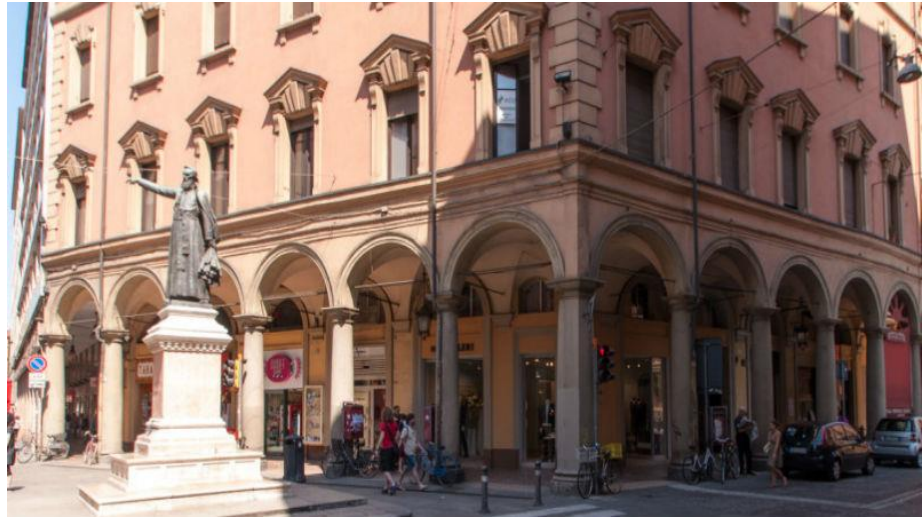
Figure 46; Via Ugo Bassi
